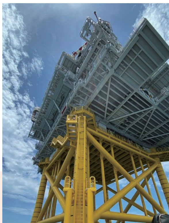
© OSHA conducted a labor inspection at Taiwan's first offshore transformer sub-station.
