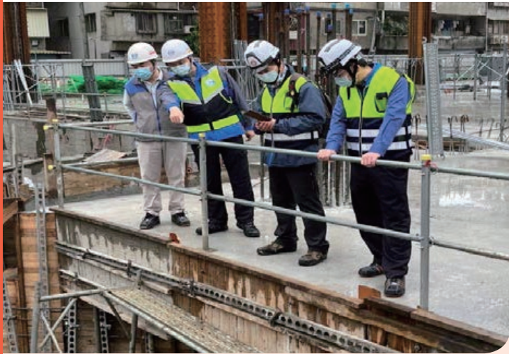
© A labor inspection at a construction site.
