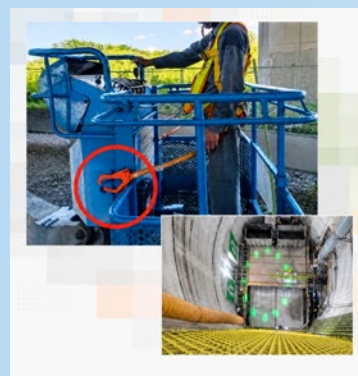
© Visible Safety Range for Full-Body Harness Hooks and Lifting Operations.
