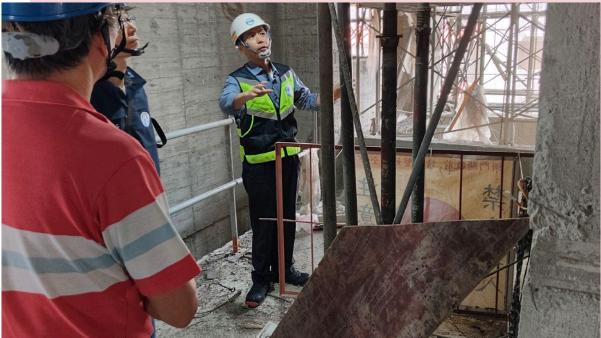
© OSHA Director-General Lin Yu-Tang led a team in conducting a labor inspection at a construction site.
