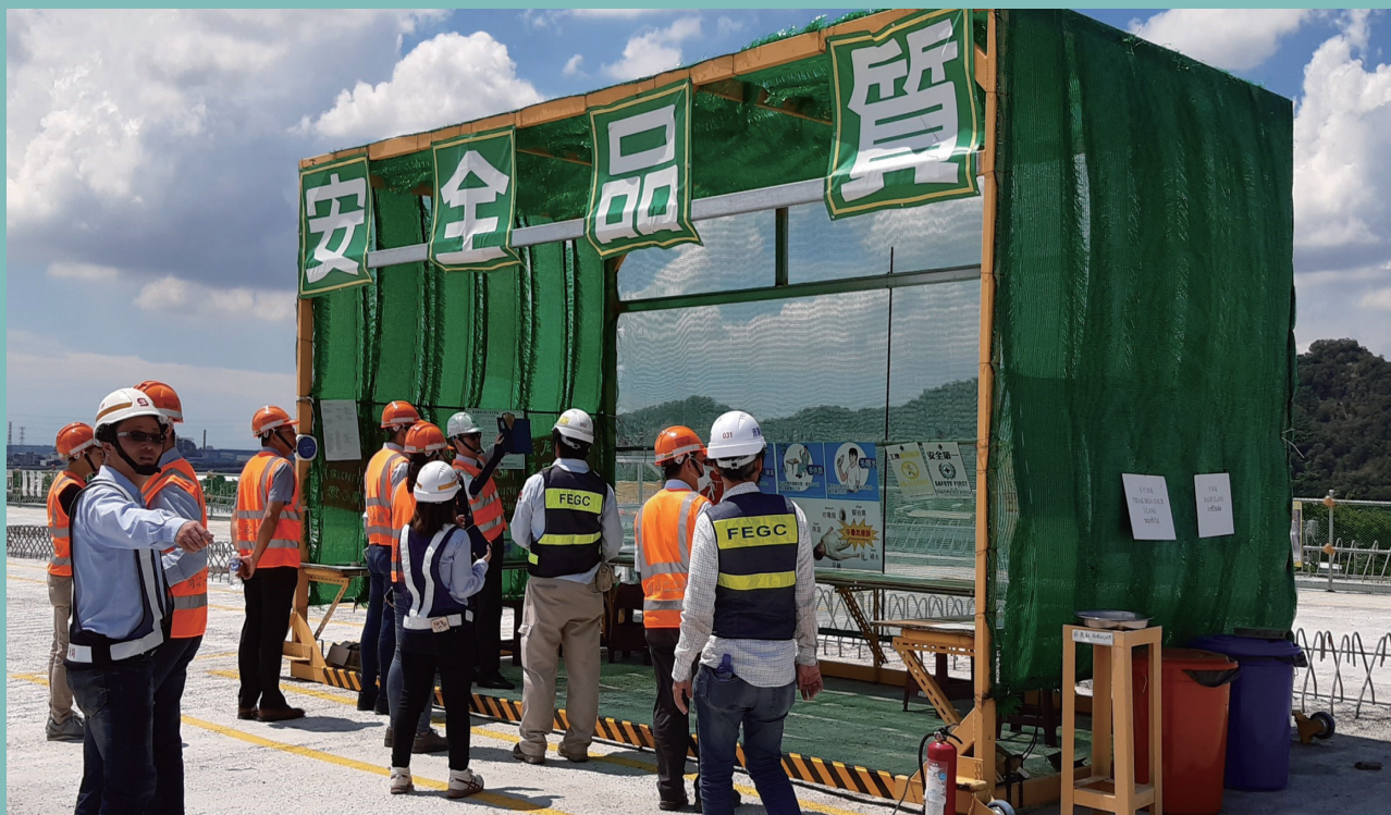
Setting up of a shaded area at a high-temperature outdoor workplace.
