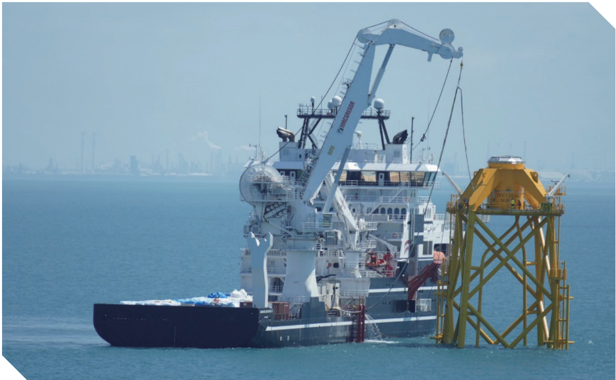
At-sea assembly of jacket foundations.
