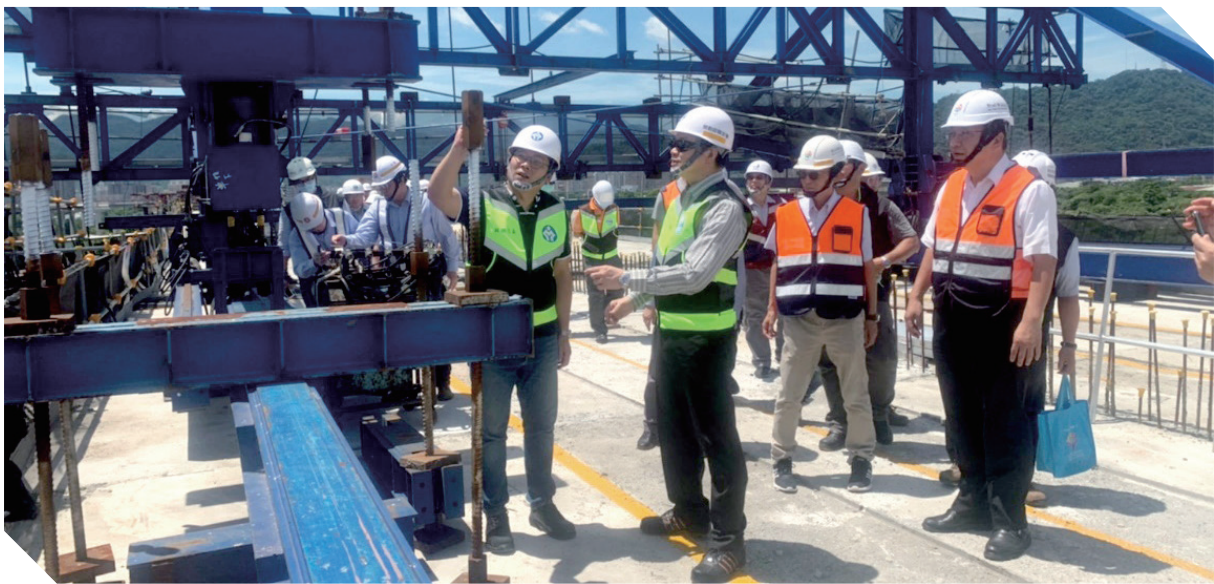
On-site inspection at a Mass Rapid Transit system job site.
