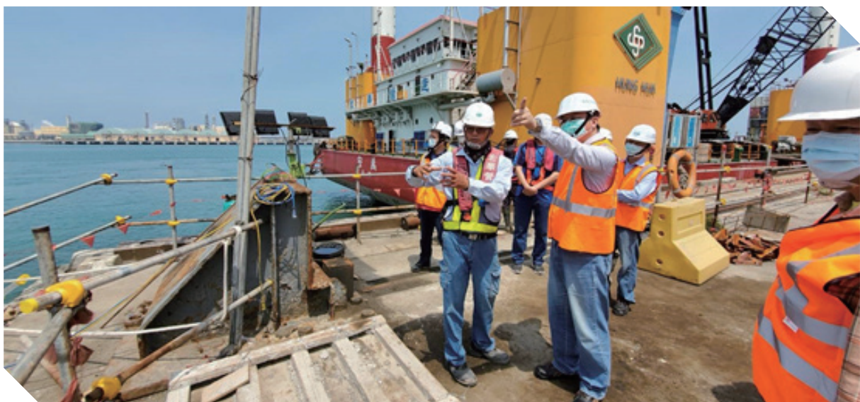
On-site inspection at a new construction site.
